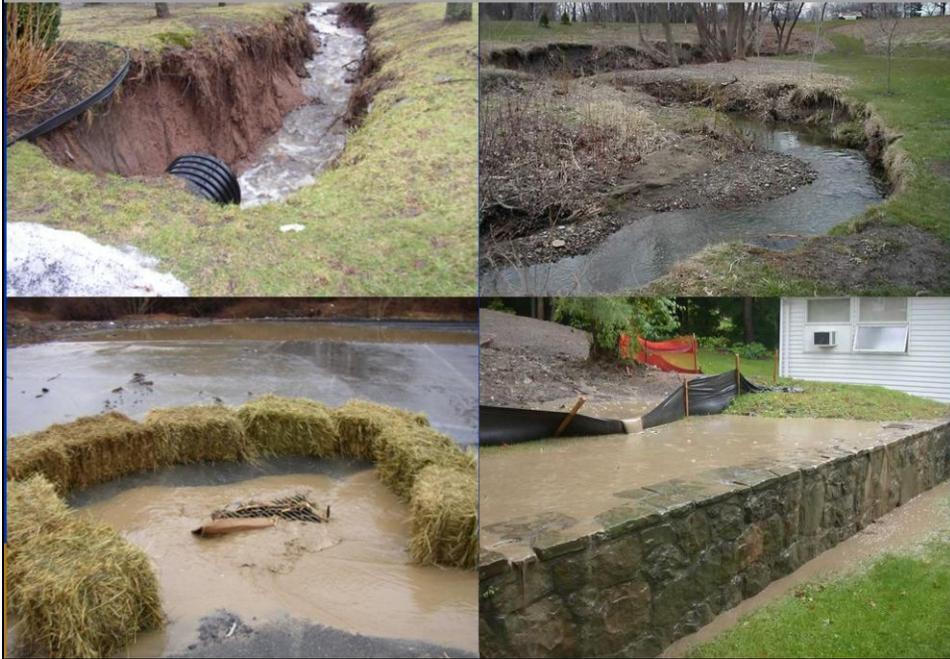
The first two pictures demonstrate the potential for stream bank erosion due to high flow. In the left side, you can see the pipe depositing water into the stream channel. The bottom two show how solids can run off from barren sites, particularly construction sites, and into water bodies. Note that in the lower left picture barrier of hay bales has been placed to filter sediment. However, the system is obviously failing.
